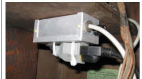
For safety's sake - a three-wire cord and fuse box installed in a Stromberg Carlson 63 console radio.
