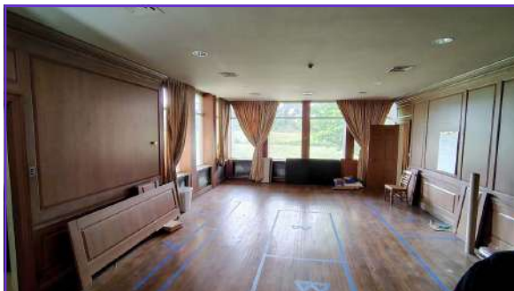
David Sarnoff's former office. The wood is being removed to be used elsewhere in the library, as this will soon become a "wet" laboratory.
